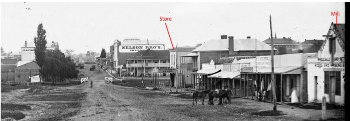
Henry Curran's Store and Flour Mill, Summer Street Orange – 1870s (State Library of NSW)
